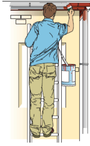
Maintaining 3 points of contact
