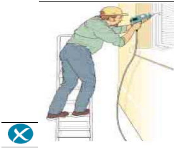
Incorrect – steps side on to work activity
